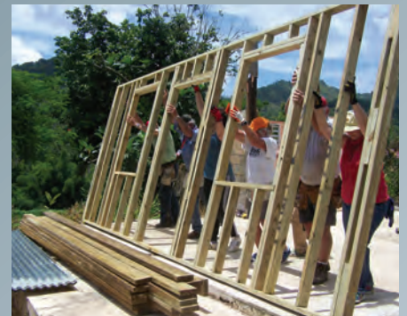
Raising a wall
