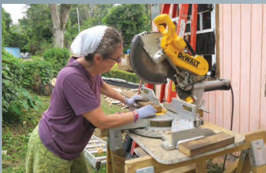
Rebuilding a home
