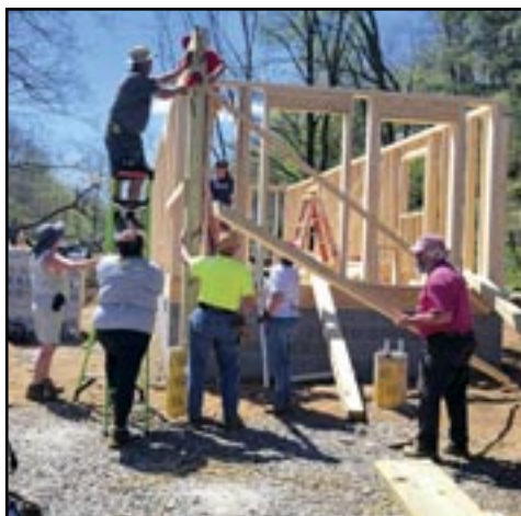
BDM volunteers work on the new house for a couple who both use wheelchairs, whose trailer home in West Jefferson, N.C., was damaged and so full of mold due to Hurricane Helene that it had to be torn down. Photo by Jim Hollen
