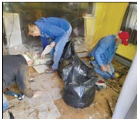
One of the four homes that BDM volunteers repaired during the one-week short-term project in Westernport, Md. These homes were damaged one year ago during a flood. Photo by Jim Hollen
