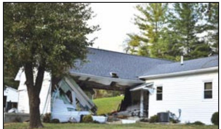
This house was one of thousands destroyed in western North Carolina during Hurricane Helene in 2024.
