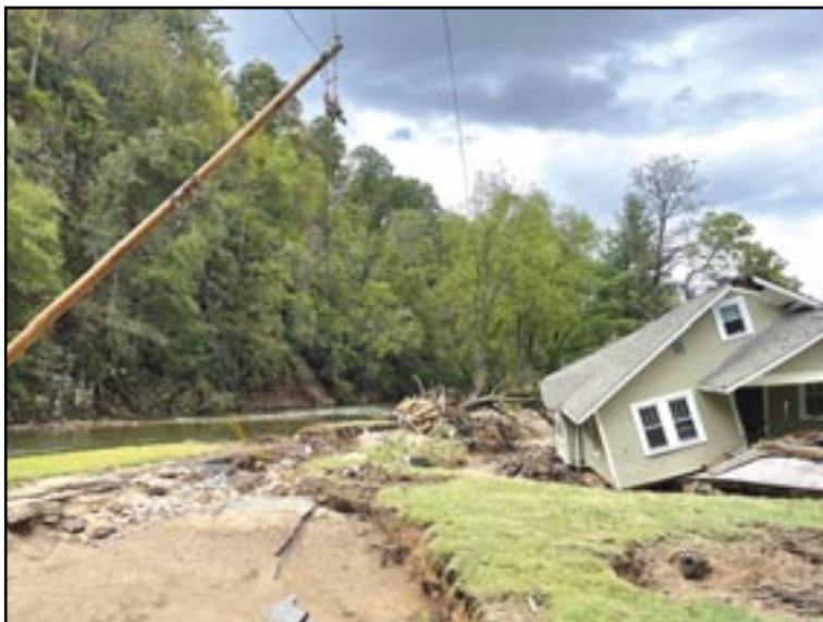
This house in southwest Virginia was moved off its foundation and destroyed due to floodwaters caused by Hurricane Helene.
