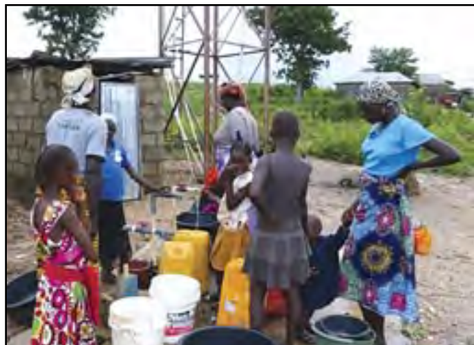
Residents of the Luvu IDP Camp in Nasarawa State, Nigeria, draw clean water from an EYN borehole.
