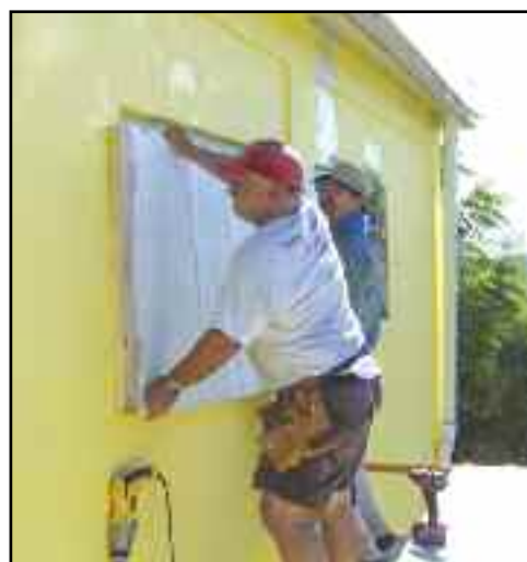
BDM volunteers painted the exterior and installed storm shutters on this St. Thomas (USVI) home in December 2018.
